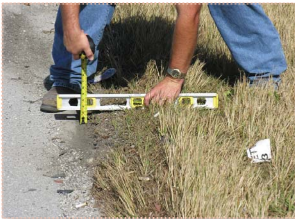
An ICA employee measures shoulder build-up for MRP compliance
