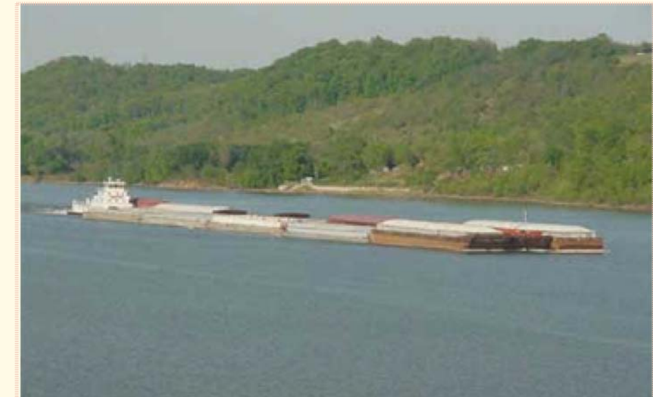
The Meade County Riverport Authority project will establish a regional port facility on a 50-acre site east of Brandenburg, KY on the Ohio River.
